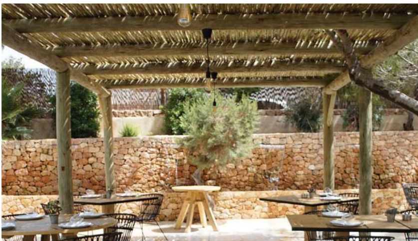
Garden hut completely formed by South African eucalyptus, autoclave treated for outdoor use
